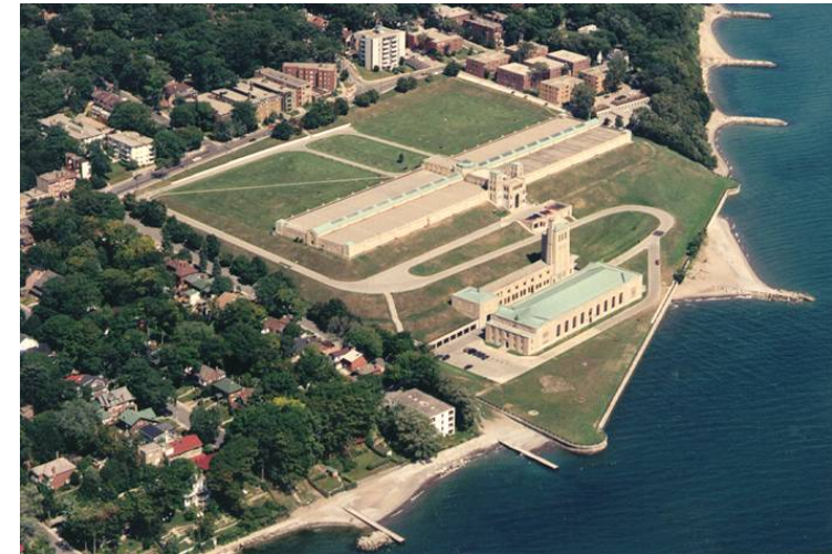
R.C. Harris Water Treatment Plant
