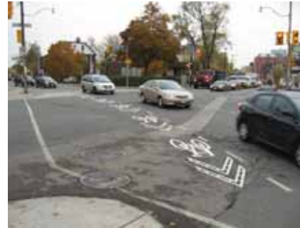
Existing treatment at Annette-Dupont.
