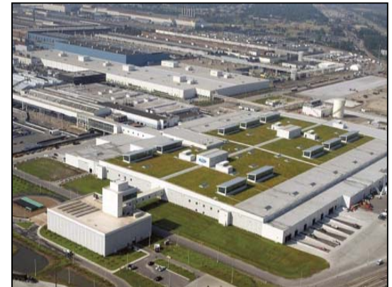
Ford truck assembly plant in Dearborn, Michigan. Recognized in 2004 by Guinness World Records as world's largest green roof (454,000 sq feet). Wm McDonough & Partners, ARCADIS Photos courtesy of www.greenroofs.org
