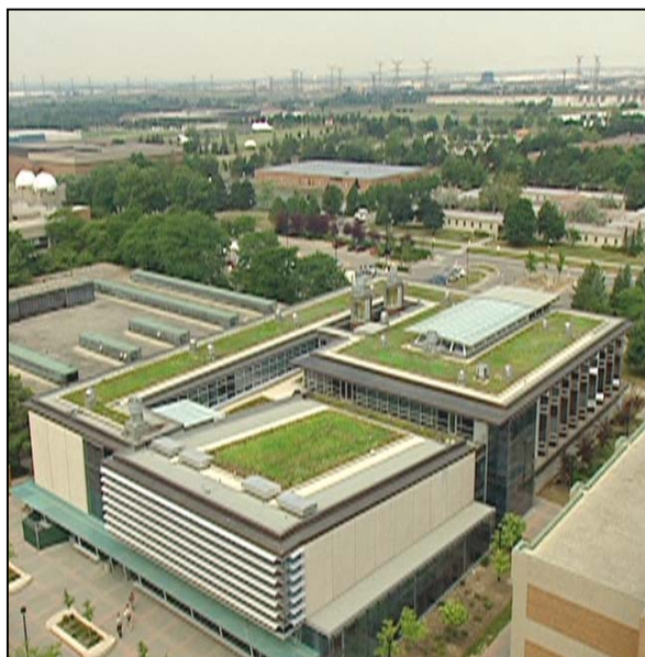
York University Computer Science Building's green roof (10% slope) Source: Green Roofs for Healthy Cities www.greenroofs.org
