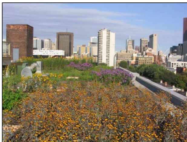
215 Spadina Avenue (Extensive green roof, 5 inches deep) urbanspace PROPERTY Group
