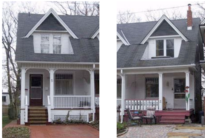
Figure 18. Like the structure above 5 and 3 Balmy Avenue
