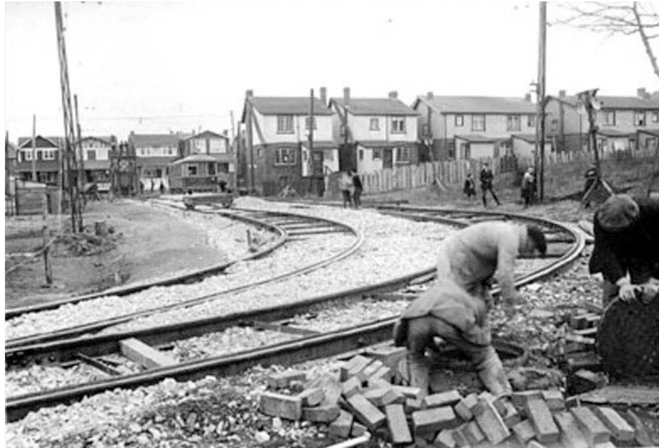
Figure 10. Construction of the Bingham Loop in 1922
