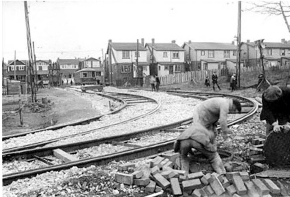
Figure 10. Construction of the Bingham Loop in 1922
