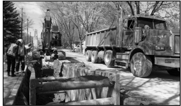
Example open-cut construction in a road
