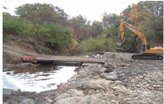
Example of construction of creek restoration
