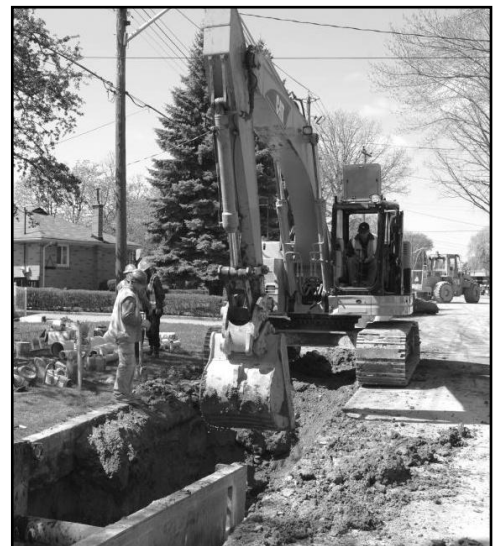
Example watermain construction
