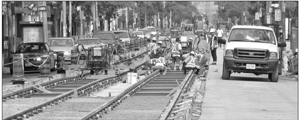
Example of TTC track reconstruction work in progress
