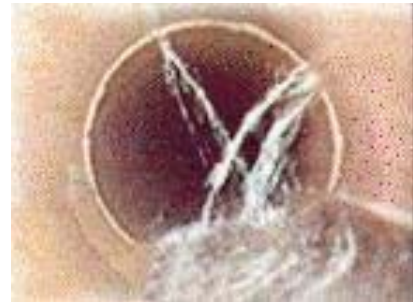
Pipe before internal grouting
