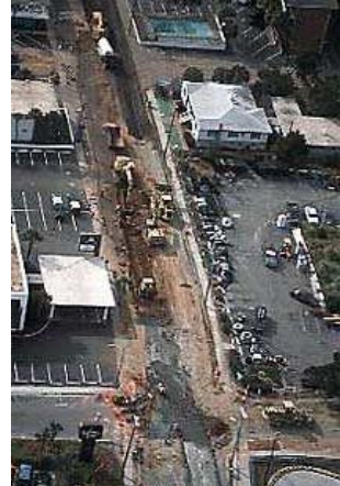
Open cut sewer replacement
