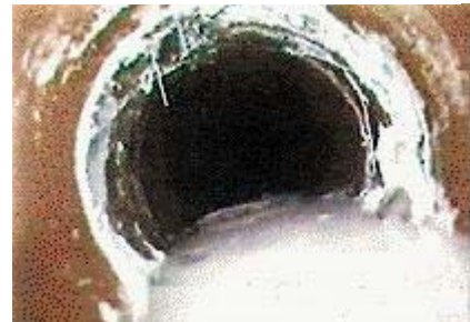
Pipe after internal grouting
