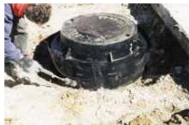
Manhole Rehabilitation
