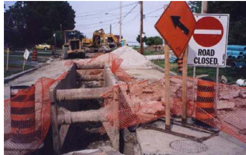
Replacement of sewer infrastructure
