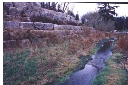
Armourstone bank protection
