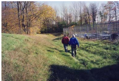
Grass swale for water conveyance and treatment
