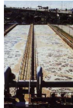
Region of Halton wastewater treatment plant modifications
