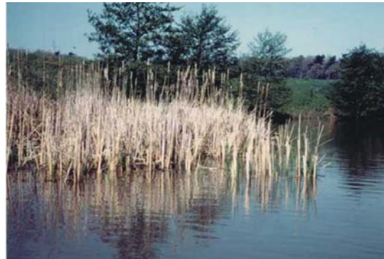
Surface storage lagoon for CSO
