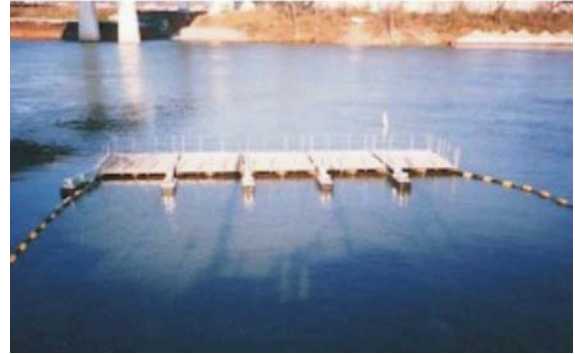
Surface baffling to trap floatable debris
