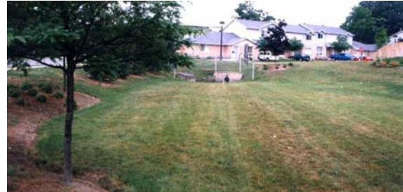
Dry pond for quantity control
