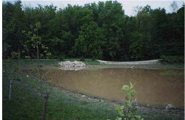
Wet pond for water quality, erosion and quantity control
