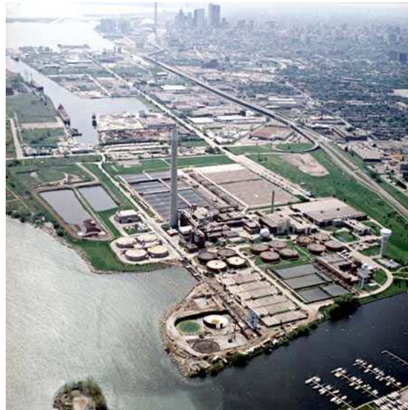
City of Toronto main wastewater treatment plant
