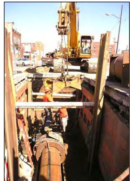
Typical Tunnel Shaft
