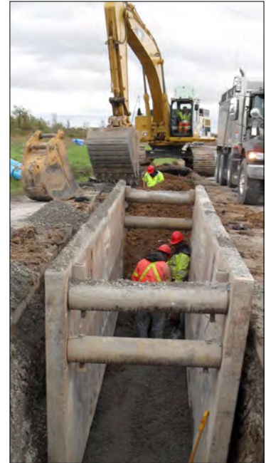
Open Cut Construction
