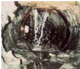
Cracked Sewer
