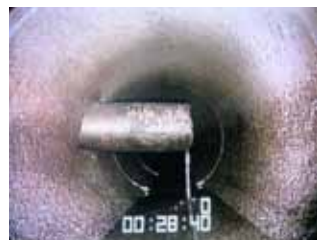
Sewer Protrusion
