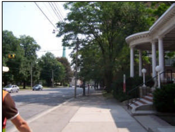
Photo 10. South view of West side of Jarvis Street at South of Carlton Street.
