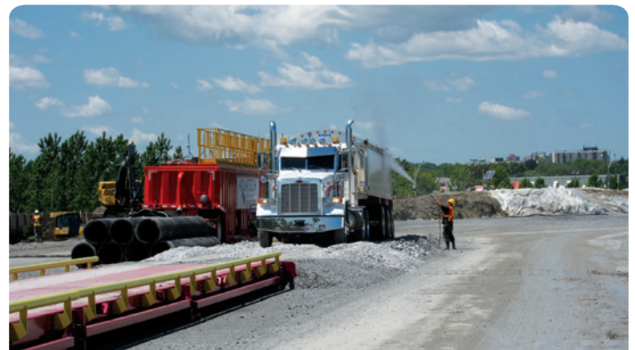
Soil Removal Operation
