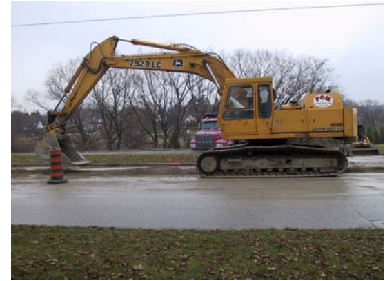
Typical On-site Backhoe
