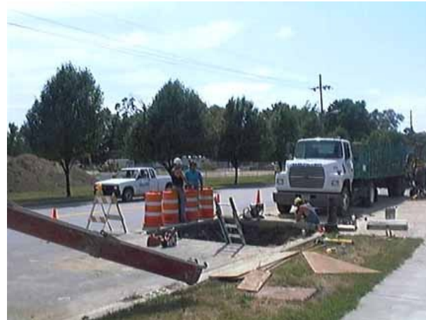
Entrance Shaft to the Tunnel Underground
