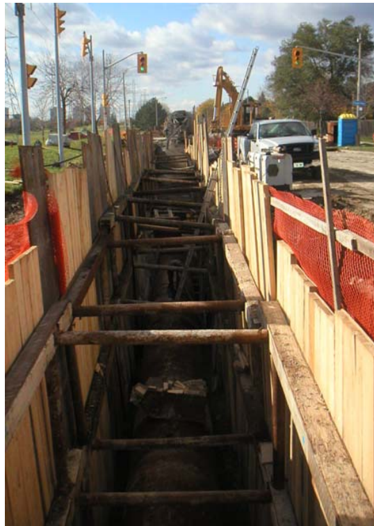
Shoring of Watermain Trench
