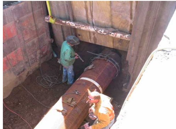
Pushing the watermain into the tunnel section
