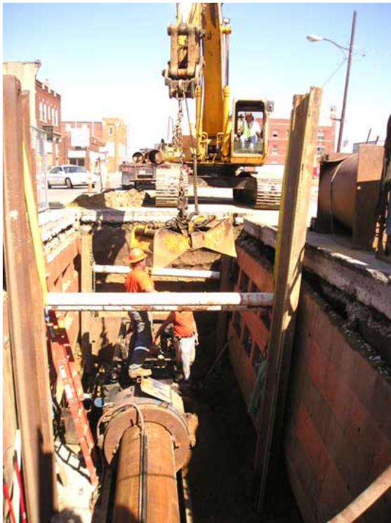
Pipe section pushed into tunnel
