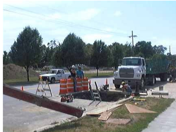
Entrance Shaft to the Tunnel Underground
