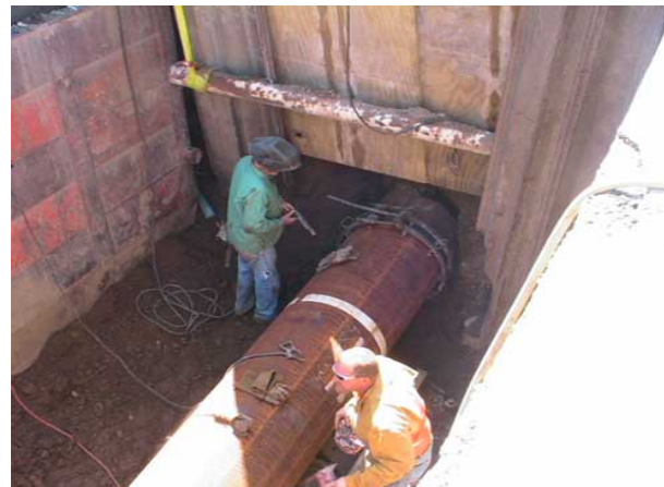
Pushing the watermain into the tunnel section
