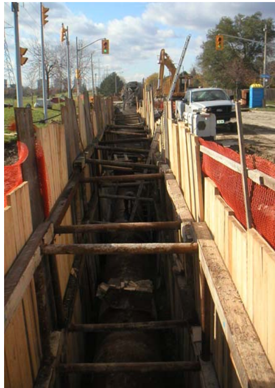
Shoring of Watermain Trench
