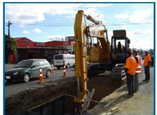
Road Sewer Separation
