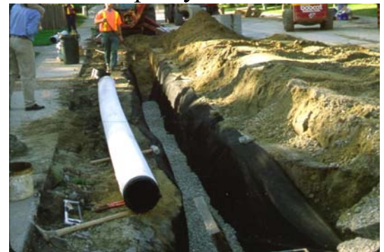
Pervious Pipe System
