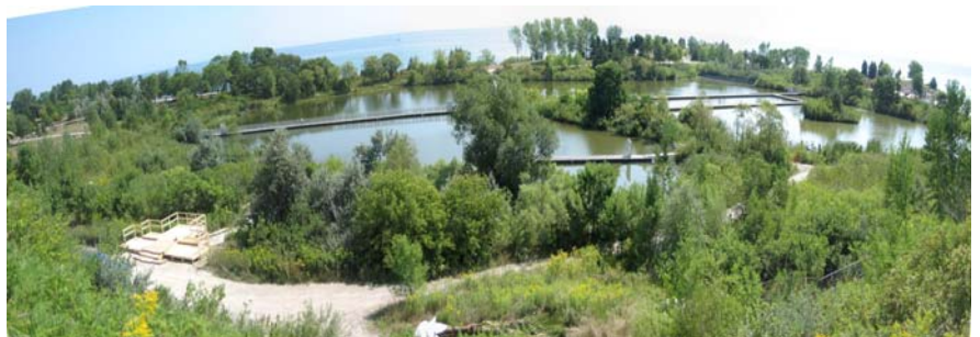
Flow Balancing Facility
