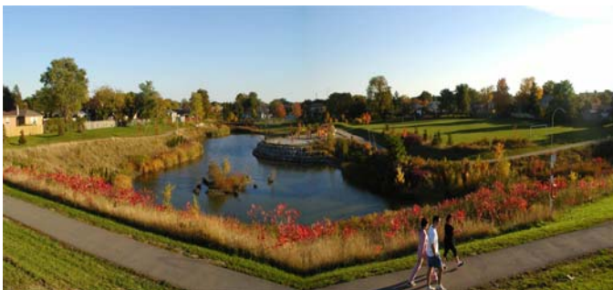
Stormwater Management Facility
