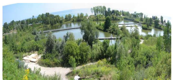
Flow Balancing Facility
