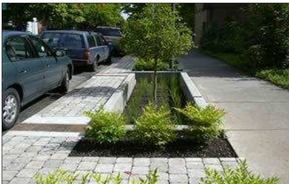
Bioretention unit in a downtown/commercial boulevard
