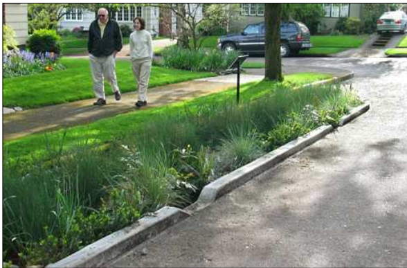
Bioretention unit on the road
