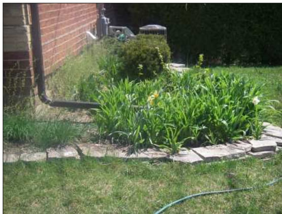
Downspout Disconnection
