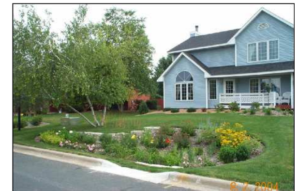
Bioretention unit within the road right-of-way
