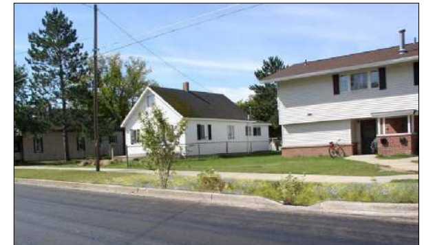
Bioretention unit within the boulevard
