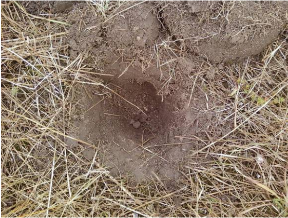
Plate 5: Example of excavated test pit (top soil mixed with gravel).
