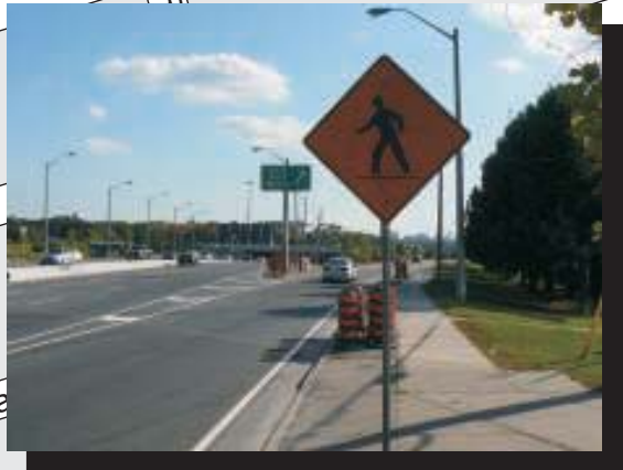
Realignment of the sidewalk and crosswalk at the Yonge St. & westbound on-ramp area.
