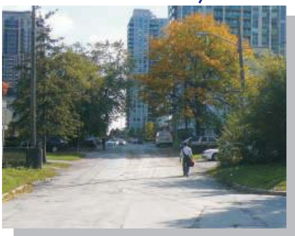
High demand pedestrian area with no sidewalks (Pictured: Bales Ave.)
