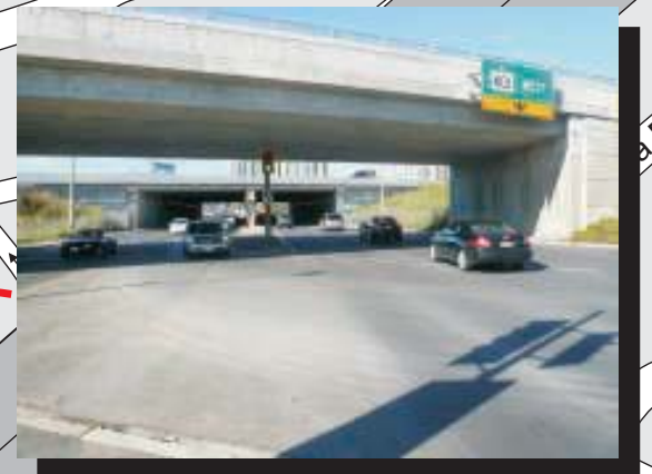
Extension of southbound left turn lane along Yonge St. at Lord Seaton Rd.
