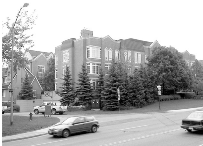
Buildings can be designed to be integrated with the local topography, hiding service areas and absorbing changes in grade
