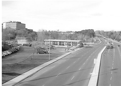
View of Leslie Street north to Sheppard Avenue from Bridge to North York General Hospital over Leslie Street
