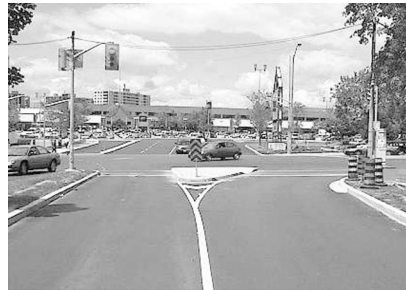
Intersection diverter prohibiting through traffic at Sheppard Avenue and Parkway Forest Drive
