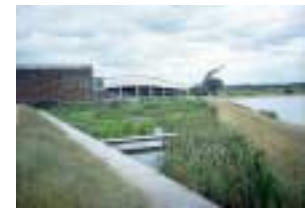
Stormwater management ponds integrated into gardens at Expo 2000 site, Hanover
