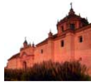
Restored Monastery of Santa Maria de las Cuevas, legacy of Seville 92
