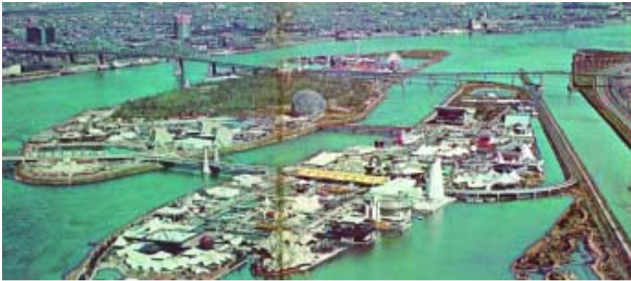
Expo 67 Aerial View
