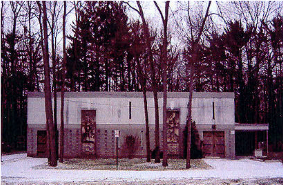
Building 191 Front (East) Elevation
