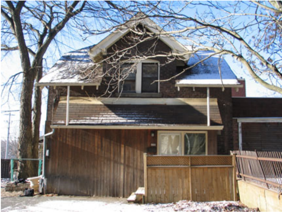
Coach House – East elevation (Broadview Avenue)
