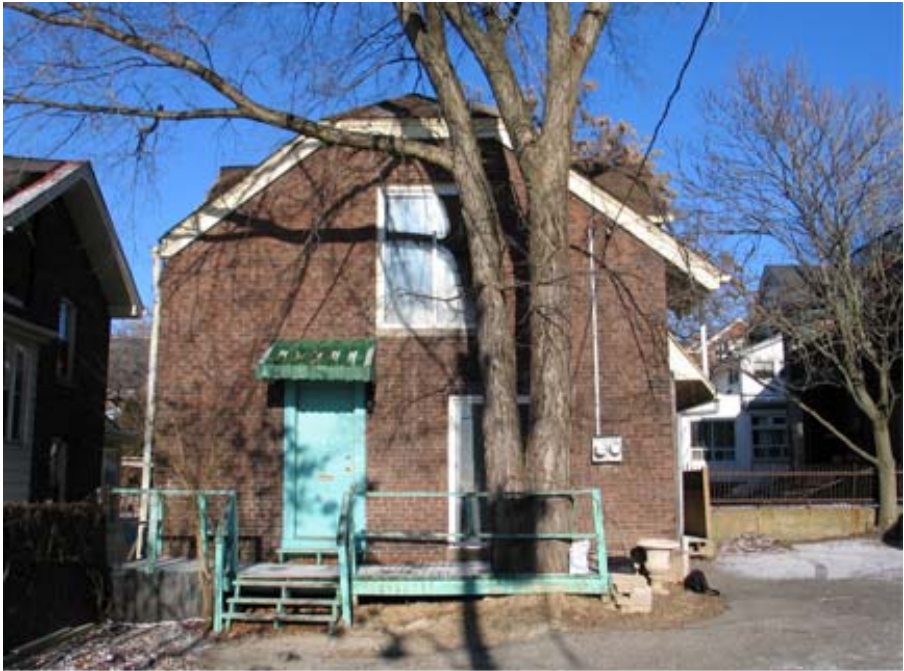
Coach House – South elevation (Montcrest Boulevard)
