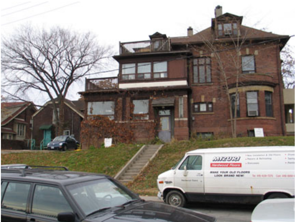
South Elevation – Montcrest Boulevard
