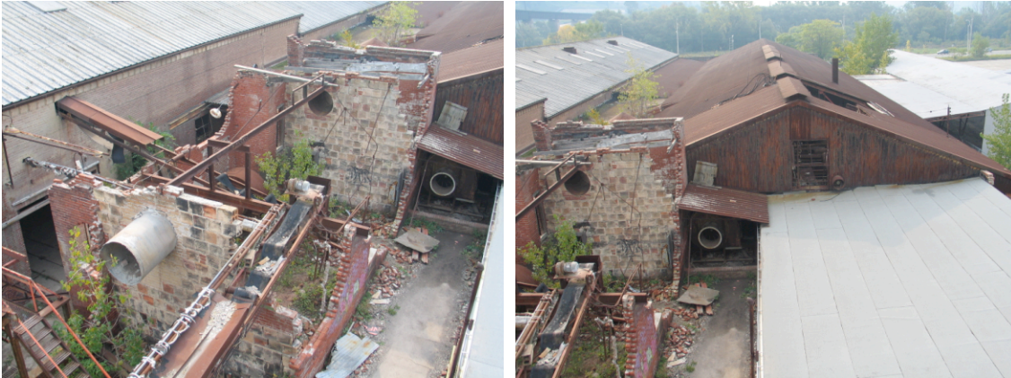
Views into Building 11B and 11C and looking south to Building 14
