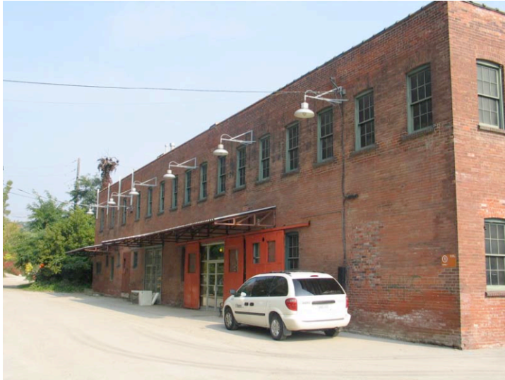
View of west elevation, 2005
