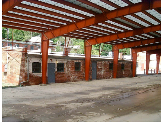
View of east elevation, 2005
