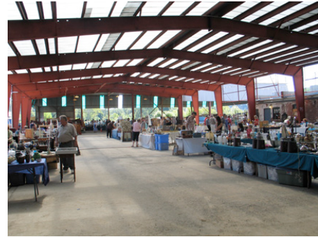
Interior view of Buildings 6 and 7, 2005
