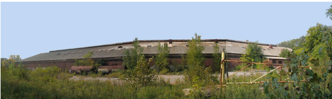
East elevation of Building 16, 2005
