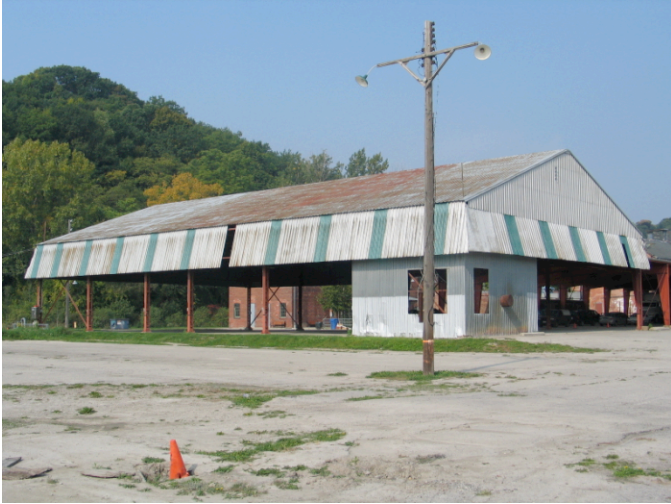
View of south and east elevations of Building 8, 2005
