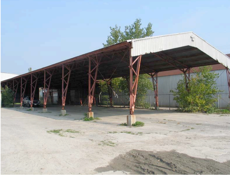
South and west elevations of Building 13
