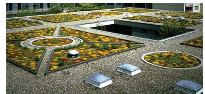
Figure 33 Photo of Green Roof, Chicago City Hall, Chicago
