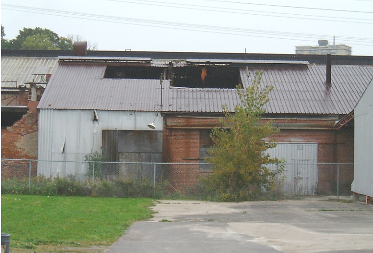
North section of Building 14 adjacent to Buildings 11B and 11C
