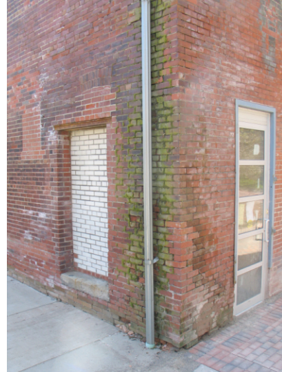
Water damage at northeast corner
