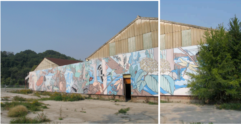
View of south elevation of Buildings 14 and 15, 2005
