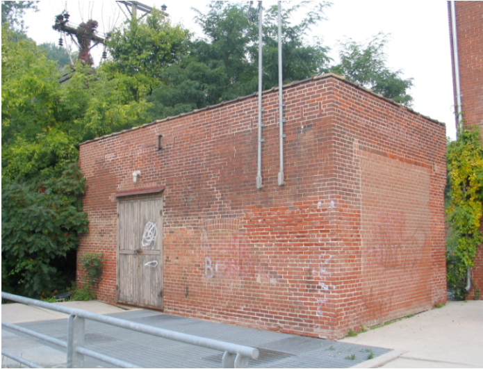
View of south and east elevations, 2005
