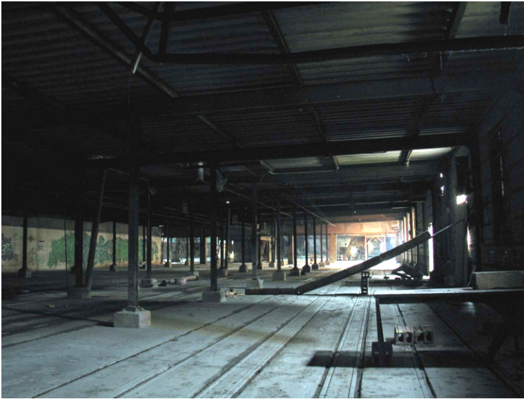
View facing south in Building 12
