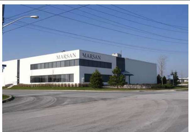
Marsan Foods Ltd. Large Industrial with Accessory Office Facility Food Research, Manufacturing and Administration Thermos Rd., Southwest Scarborough Employment District
