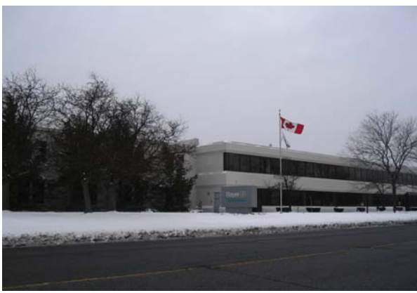
Bayer HealthCare Canada Large Bio-Tech Facility Biotechnical Research and Manufacturing Rexdale Employment District
