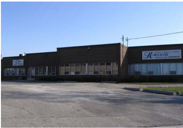
Old Industrial Multiple Continental Place, Southwest Scarborough Employment District
