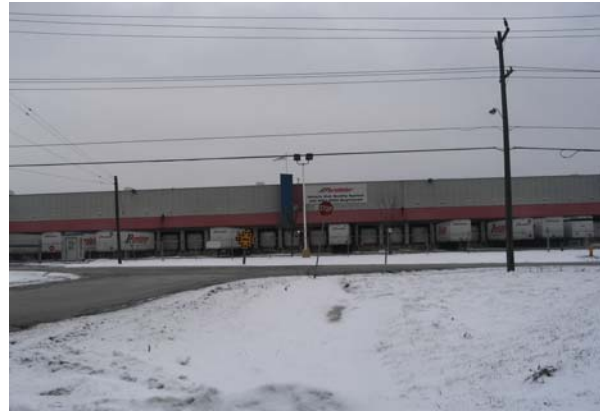
Purolator Courier Ltd. Package Sorting and Distribution Rexdale Employment District
