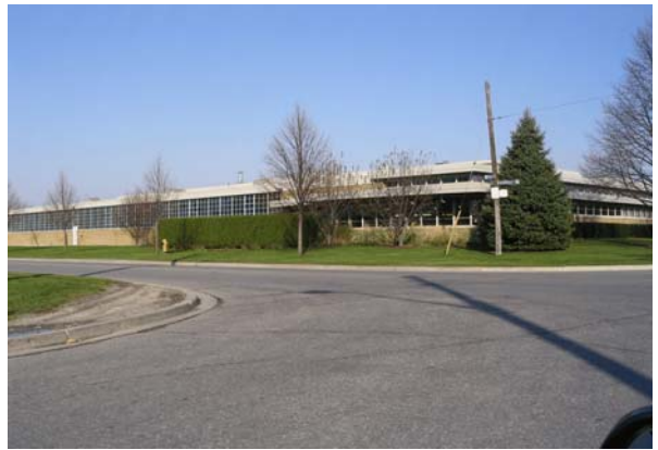
Large Older Industrial Facility Southwest Scarborough Employment District
