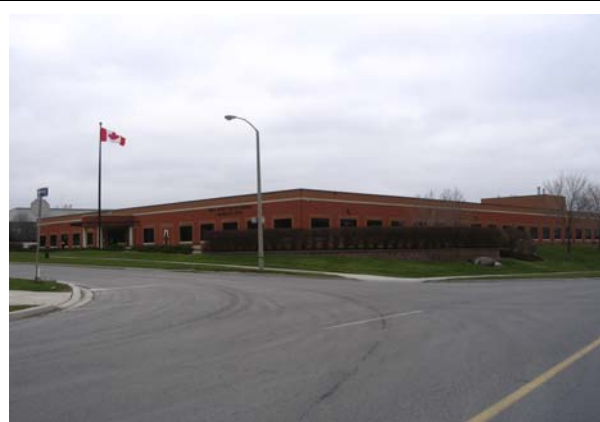
Large Newer Industrial Facility Tapscott Employment District
