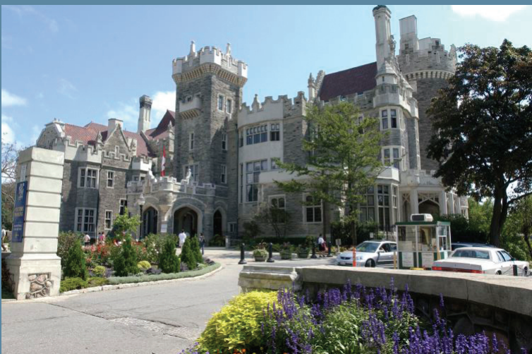
Above: The stables at Casa Loma after partial restoration work
