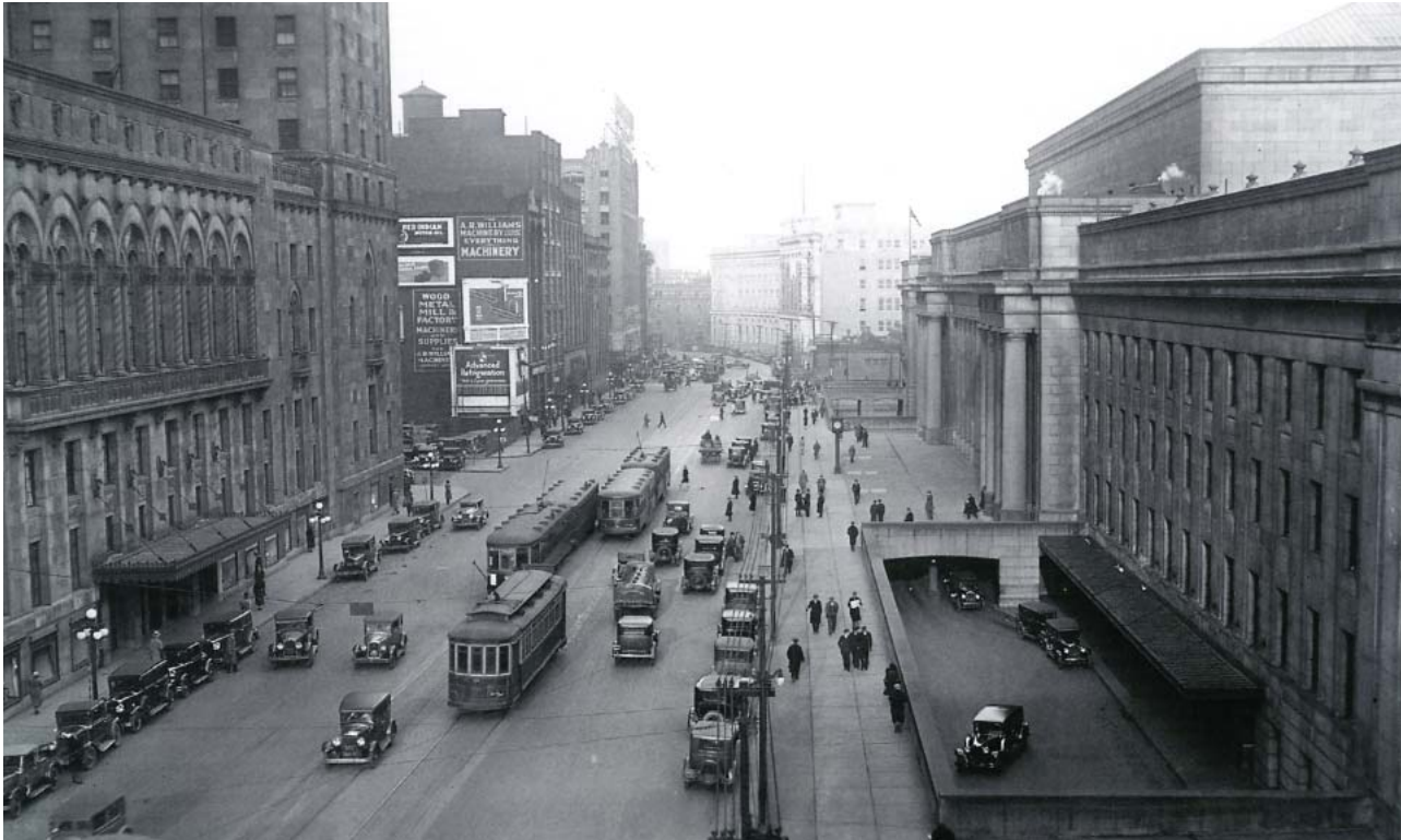
Front Street looking east at Union Station and the Royal York Hotel (1931). This view shows the clarity of the relationship of Union Station and the Royal York Hotel. Even though pedestrian demand has increased dramatically, the amount of sidewalk space available today is not significantly different from that provided in 1931. Note also how the lack of clutter and the absence of a median and extraneous signage clarifies the public realm.
