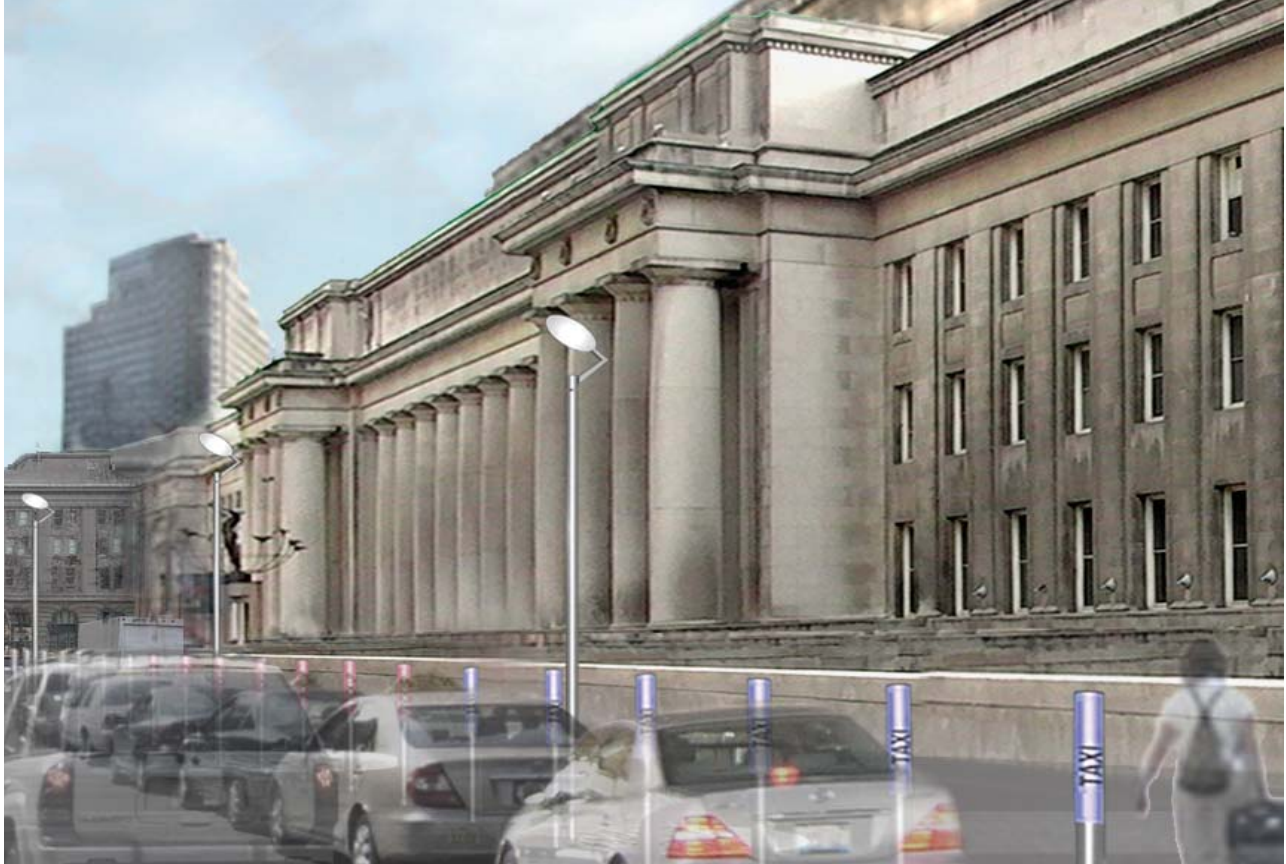
This diagram shows a designated taxi pick-up area in front of Union Station with rationalized and consolidated taxi signage. These improvements reinforce the idea of a 'pedestrian priority zone' acting as a traffic calming influence
