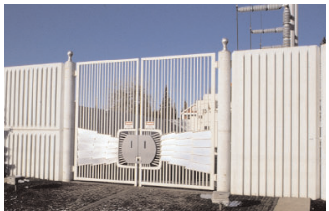
“Gate, electrical substation”, Clair Colquitt – Seattle
