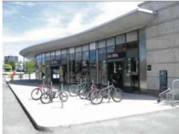
Don Mills Subway Station
