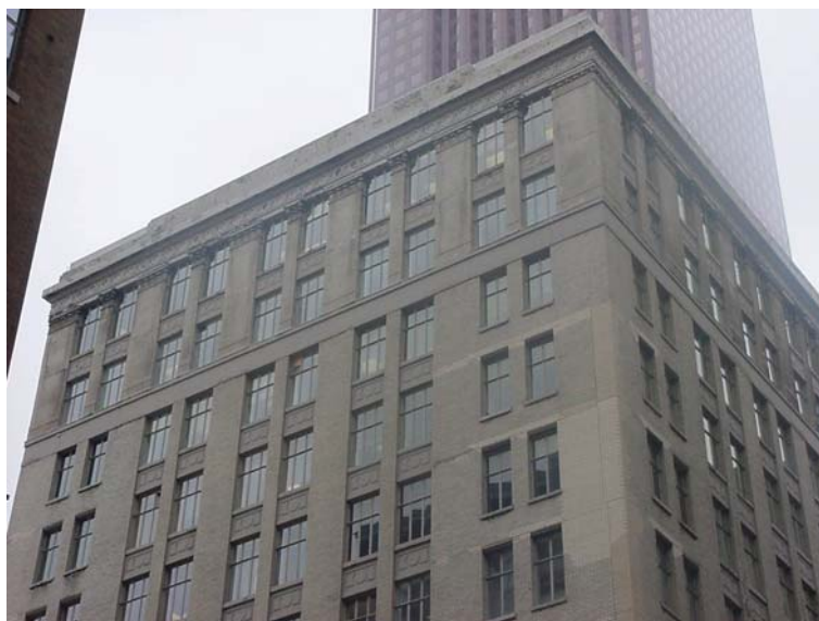
North-west Corner (Upper Capital Zone)
