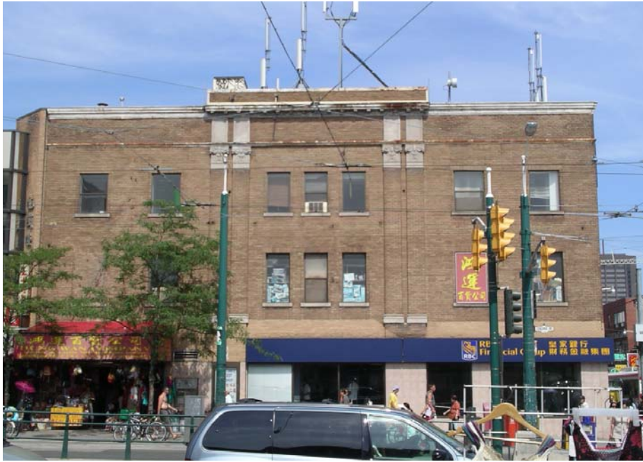
Principal (west) facade
