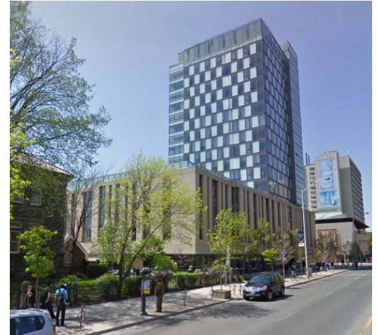
The shaft of tall buildings will have a small floorplate and be located on top of mid-rise or low-rise base buildings. The building shown above has a 4 storey base and 17 storey shaft.
