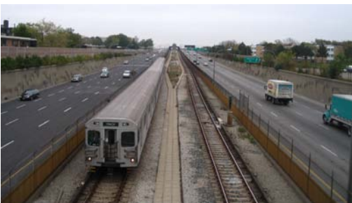
The Allen Road is a physical barrier that divides the Lawrence-Allen area.
