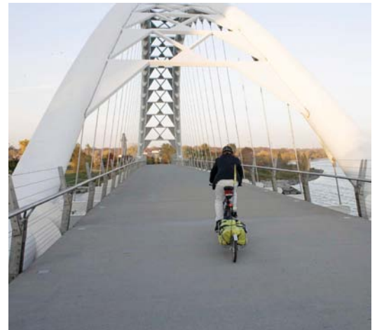
The Humber River Bicycle and Pedestrian Bridge is an example of how new bridges can help to overcome the barrier of the Allen Road, while improving the connectivity and the beauty of the neighbourhood.
