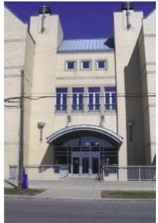
The Barbara Frum Library will be renovated to serve the growing community.
