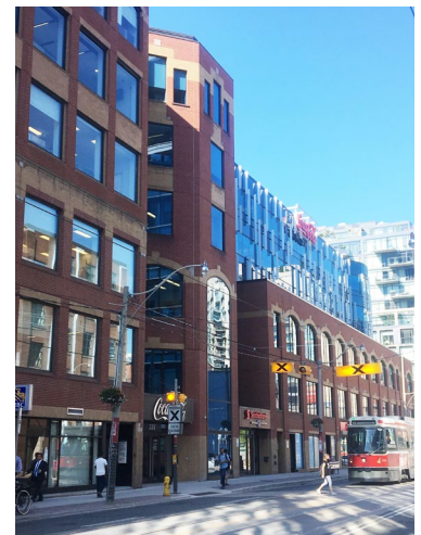
Non-residential buildings on King Street East in King-Parliament
