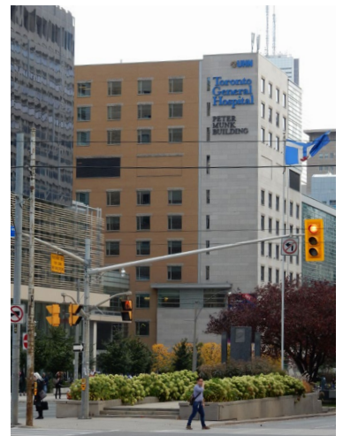
Toronto General Hospital on University Avenue
