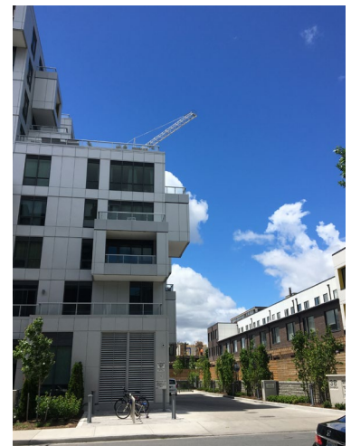
Side step-backs create a transition down in height to lower scale buildings
