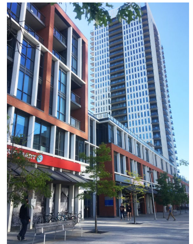
Base buildings along Regent Park Boulevard
