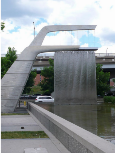
Water filtration feature at Sherbourne Commons
