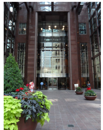
Grade-related space in front of Scotia Plaza on Adelaide Street West in the Financial District
