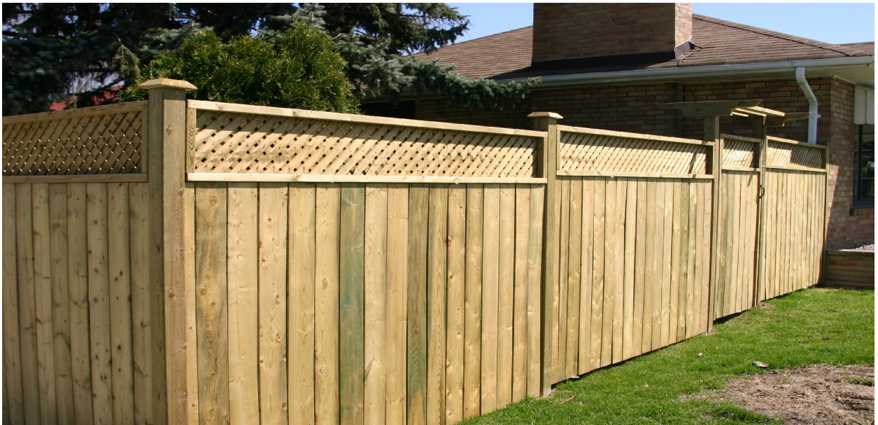
Photographs of constructed fence
