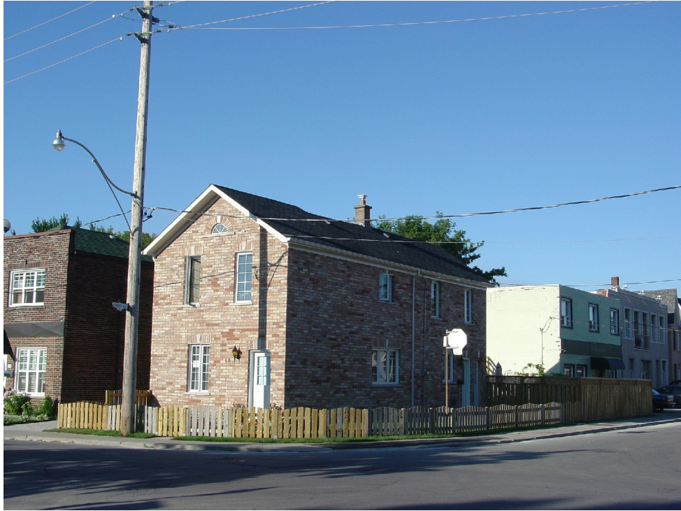
Photograph showing the property and the Fence Encroachment
