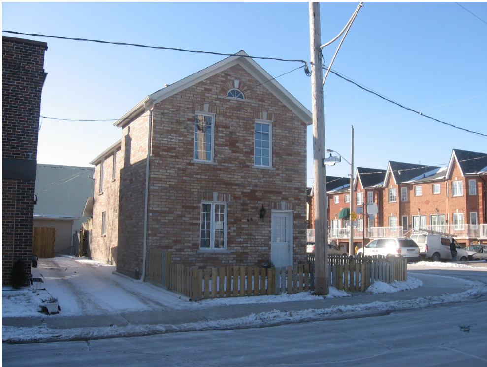
Attachment 3 – Photographs showing the Fence Encroachment
