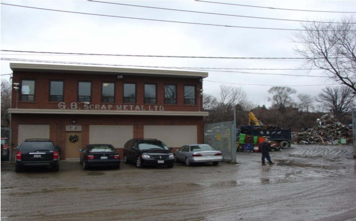
Photograph # 1 – Front Elevation of 96 Hyde Avenue
