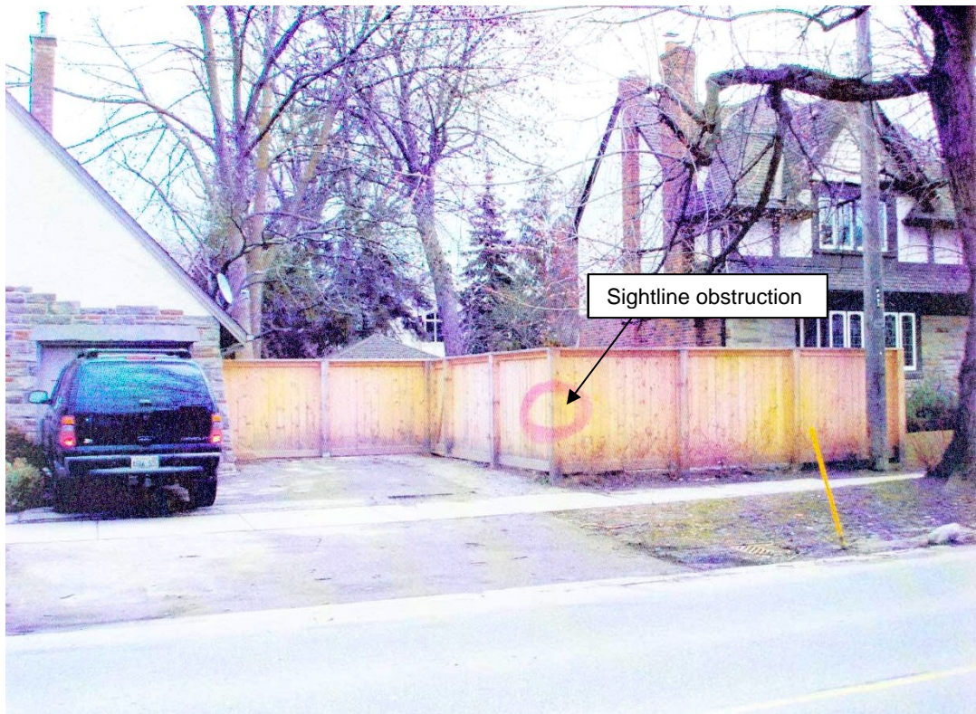
Attachment 3 – Sketch of the 1.83 metres high close board wood fence
