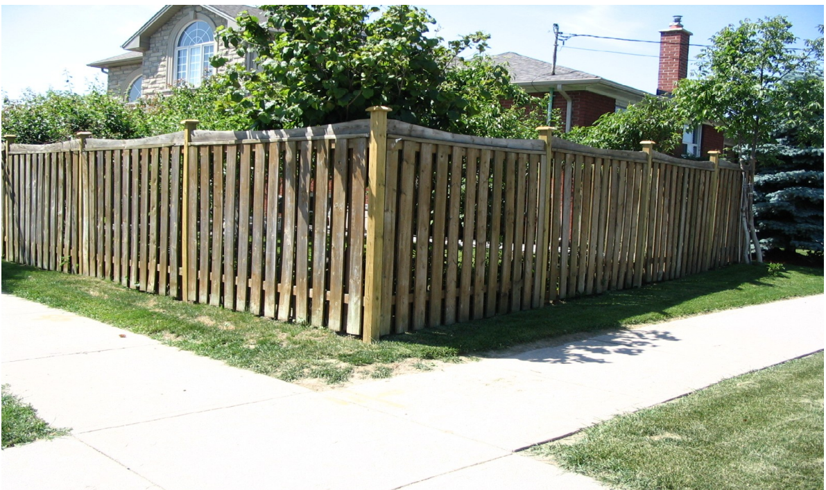
Photograph # 4 - Showing the Northeast elevations/corner as at June 11, 2007
