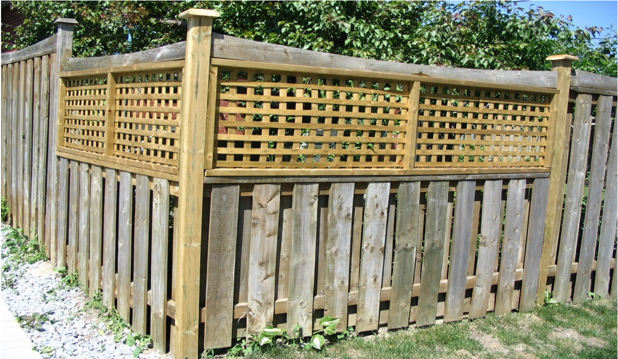
Photograph # 3 - Showing the Southeast elevations/corner as at June 11, 2007
