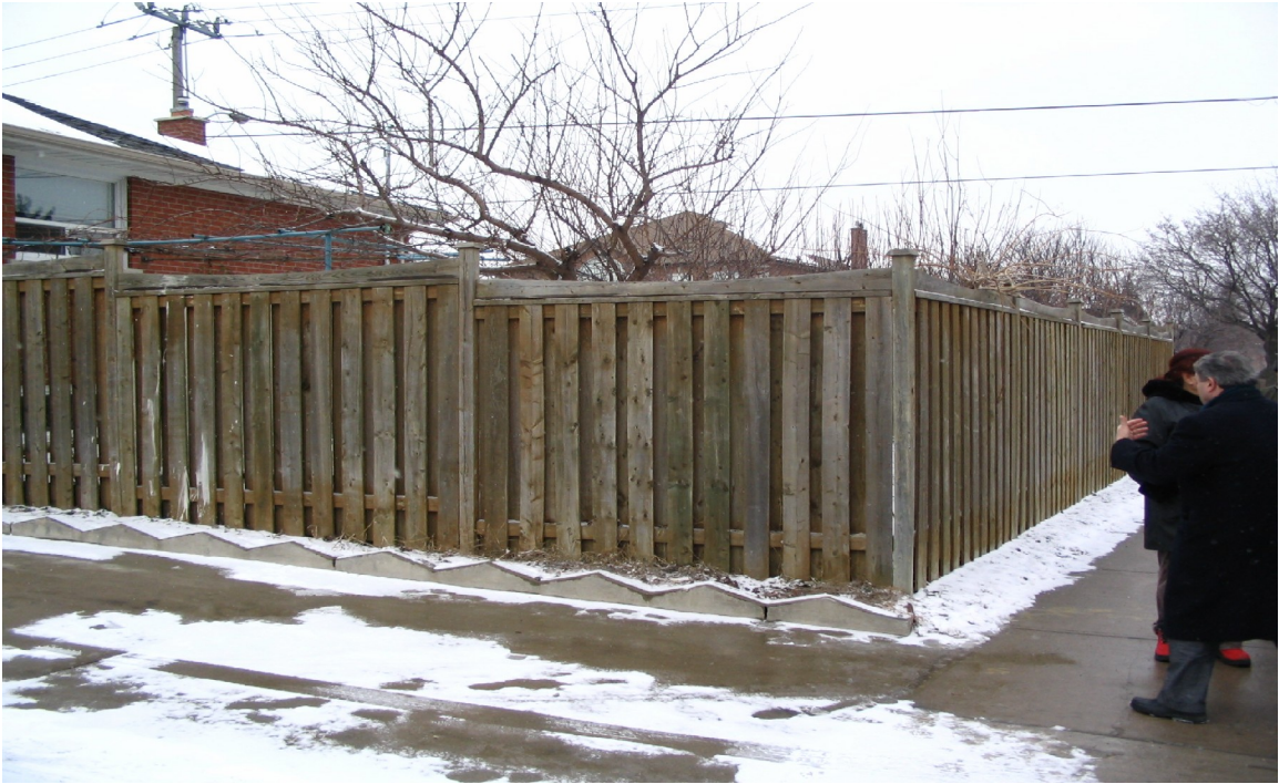
Photograph #1 - Showing the Southeast corner of the property/fencing
