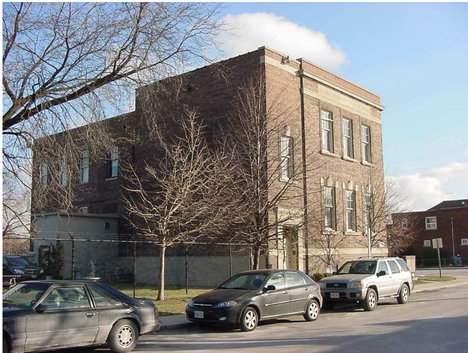
View of the north elevation and east wing (left).
