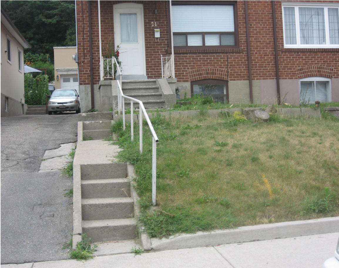
Photograph showing the proposed location of the encroachment(s) @ front elevation/yard
