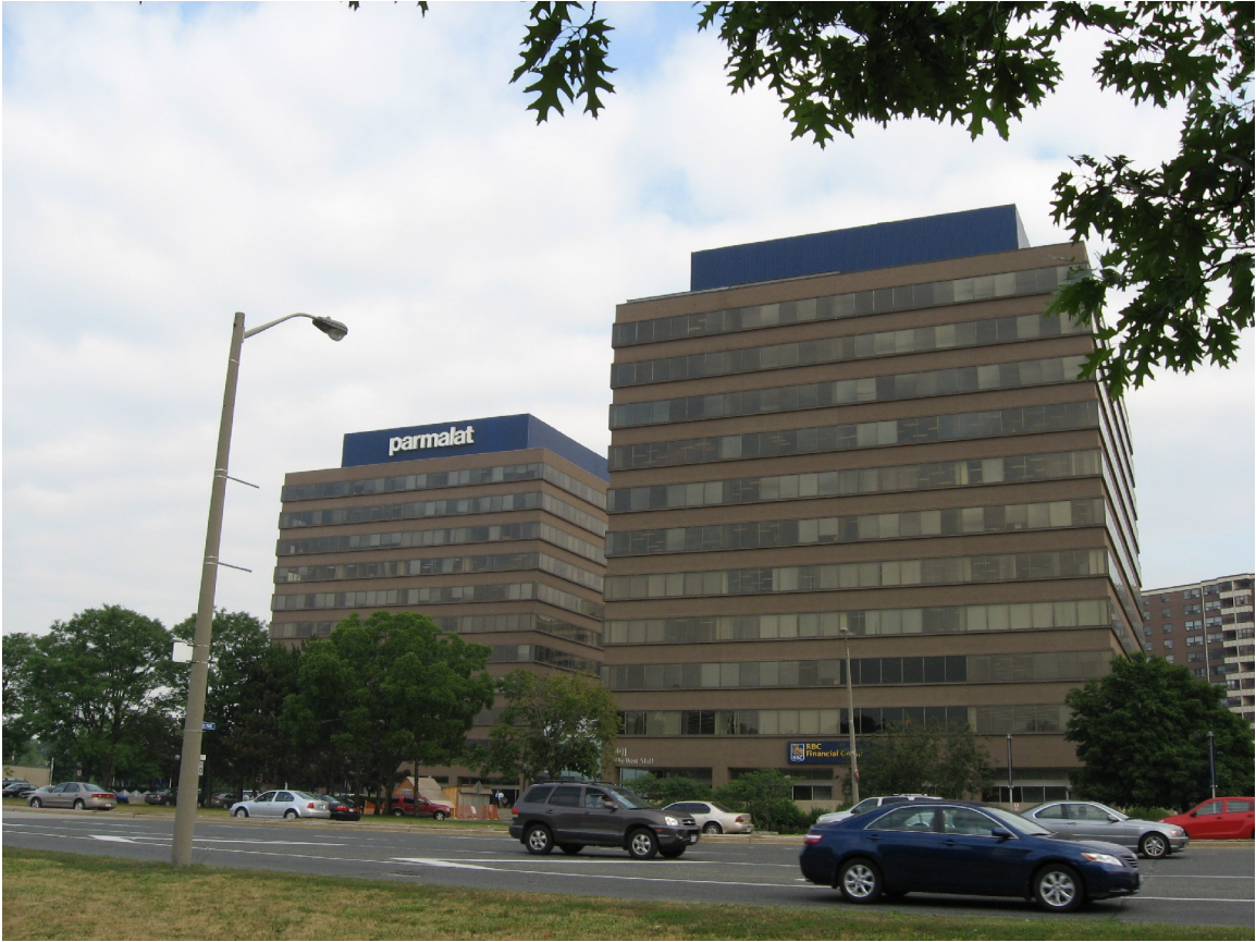
The South Elevation of 401 The West Mall
