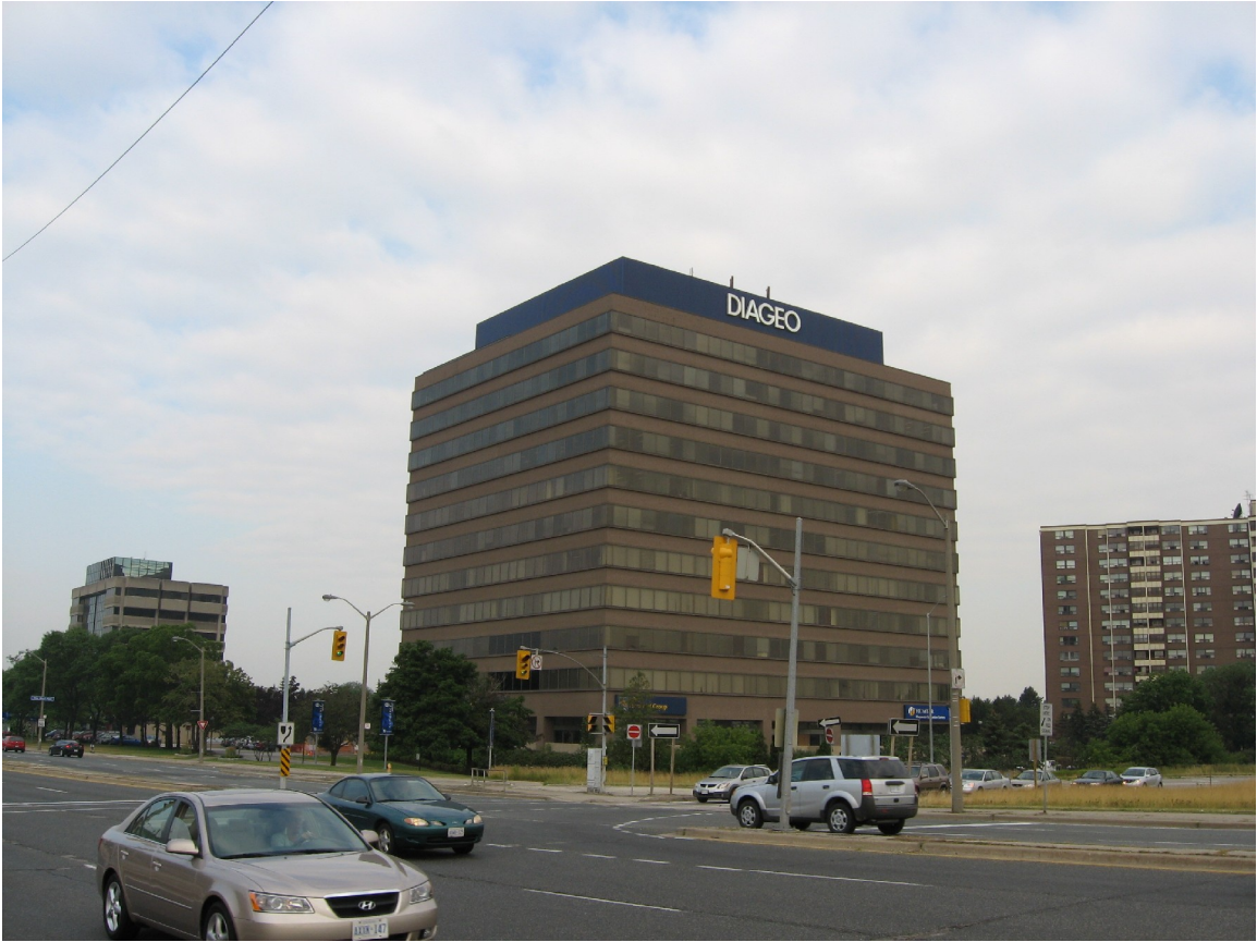
The east elevation of 401 The West Mall.
