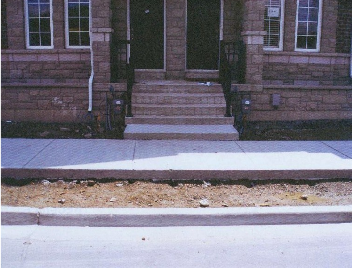
Attachment 5: Photograph showing the front entrance step and handrail
