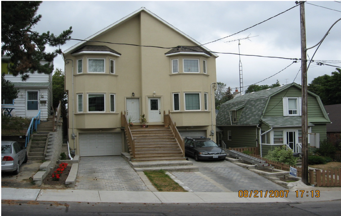
Photo 1 – Showing the front elevations of 36 and 38 Morningside Avenue
