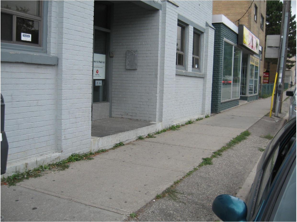
Attachment 6: Photograph of the building looking north on Islington Avenue Showing the raised front entrance step
