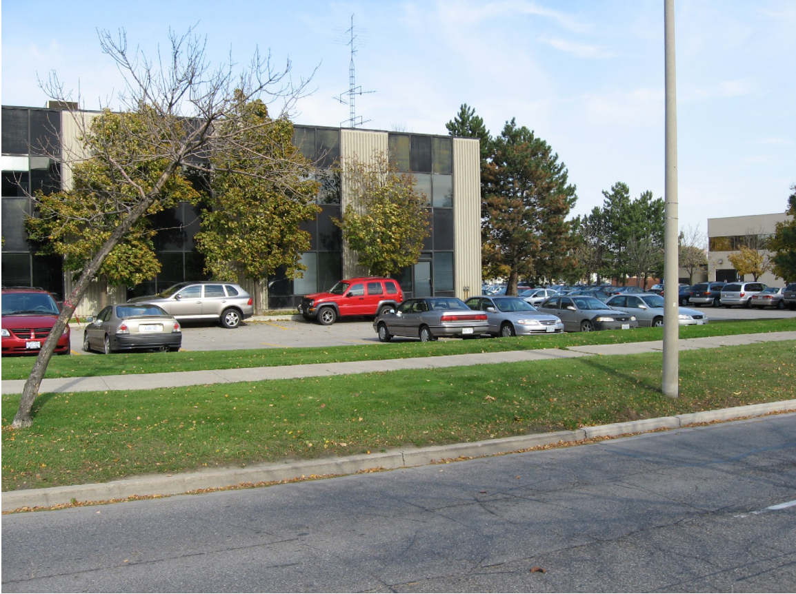
Partial west elevation of 60 International Blvd
