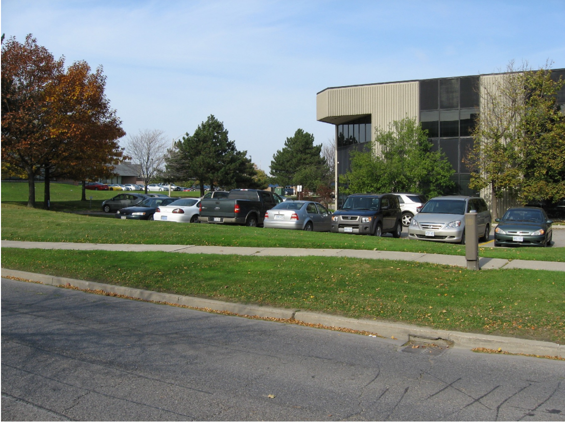
Partial west elevation of 60 International Blvd
