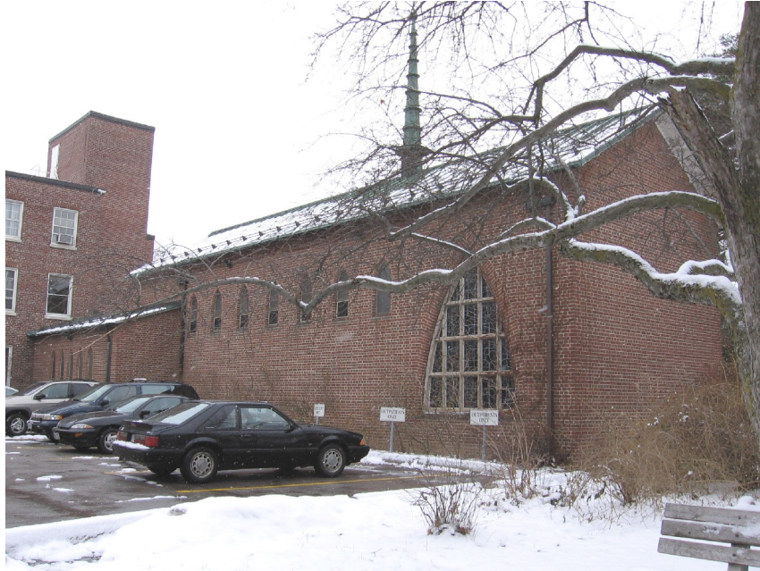
Chapel, showing east (left) and north (right) walls
